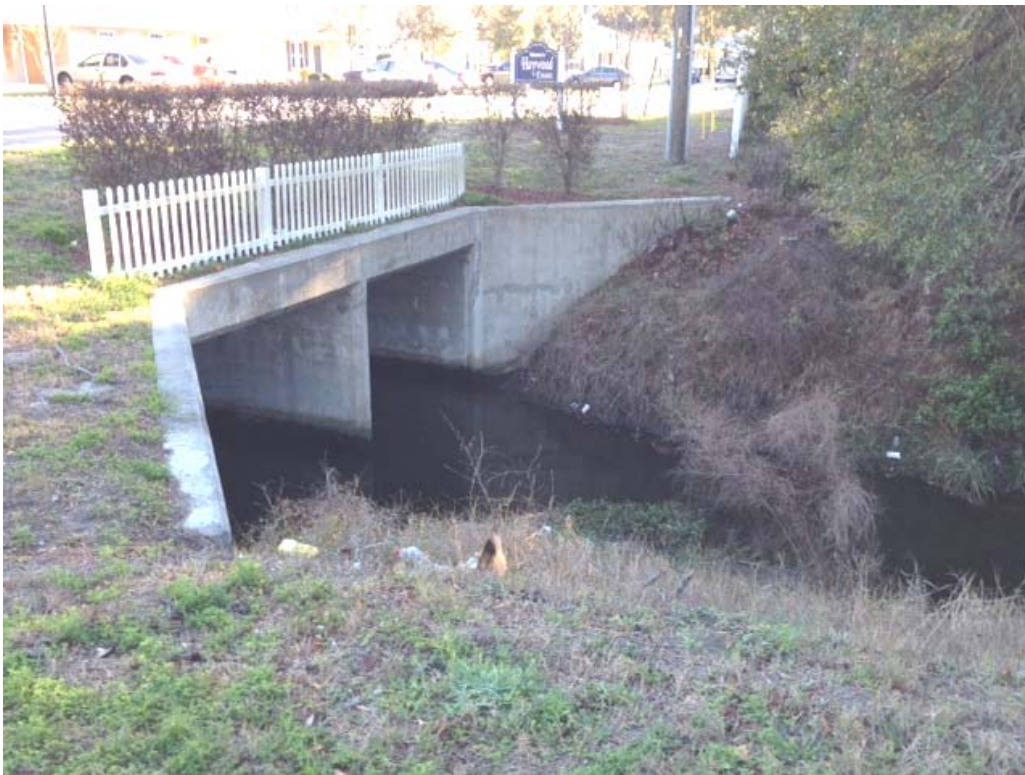
Large culvert on A1A.
